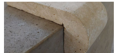
REMODELED POOL COPING
